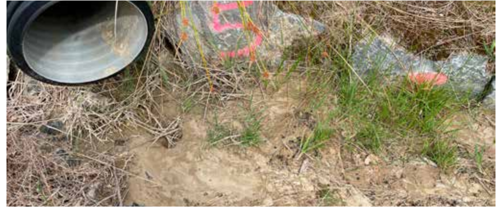
Sediment in the water table for the study site that has come from the diversion flume that takes water from a cut face above the study site.
