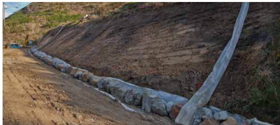
The cut face with horizontal 'scarifying' and the rock toe prior to backfilling. The plastic sheeting is a temporary flume prior to the installation of the diversion flumes.
