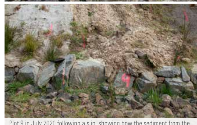
Plot 9 in July 2020 following a slip, showing how the sediment from the slip was retained on the rock toe and kept out of the water table until the material was able to be removed.
