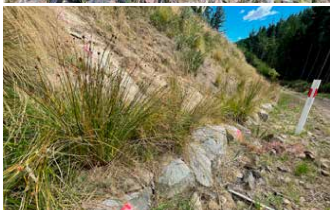
The rock toe in January 2021 showing the established vegetation that is also helping to trap any sediment that does come off the cut face.
