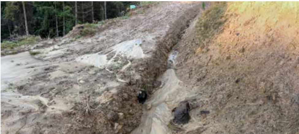
Evidence of erosion and loess runoff from cut faces and track above the study site.
